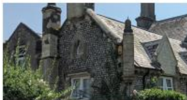
Flint work with flint chipping (galleting) to the joints
