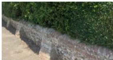
Low height flint and brick wall
