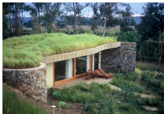
Example of a green roof
